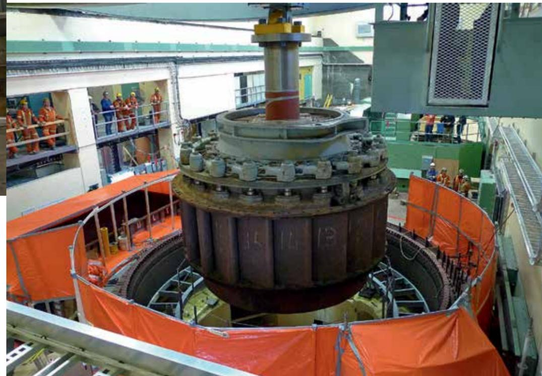
A turbine distributor is removed from the powerhouse at Rapides-des-Quinze in Quebec, Canada.
