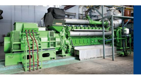
Up to ten years of service without maintenance or fatigue failure. The CT-couplings ("Compression Type"-couplings) from Voith protect the driveline of gensets against transient shock loads and vibrations. This extends the life and durability of the entire system, by ensuring a smooth and quiet operating condition. The rubber-in-compression principle is failsafe by design.
