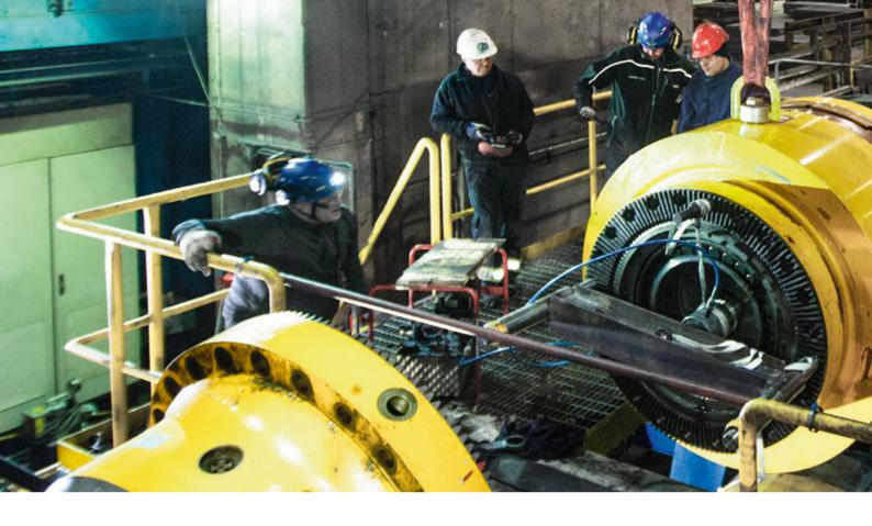
SSAB utilizes Voith torque limiting couplings to protect valuable equipment at its heavy plate mill in Oxelösund, Sweden. The Voith couplings protect the drivelines from overloads during production and therefore help ensure that the equipment works reliably and efficiently at a maximum level.
