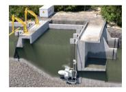
A conventional trash rack system directs the water to the StreamDiver turbine through a inclined inlet.
